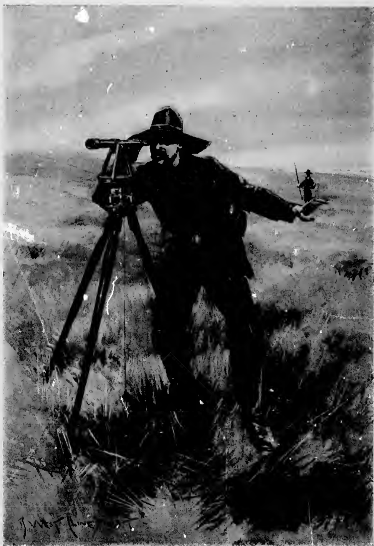
The Engineer. (Running the line with a transit on the Plains.)
