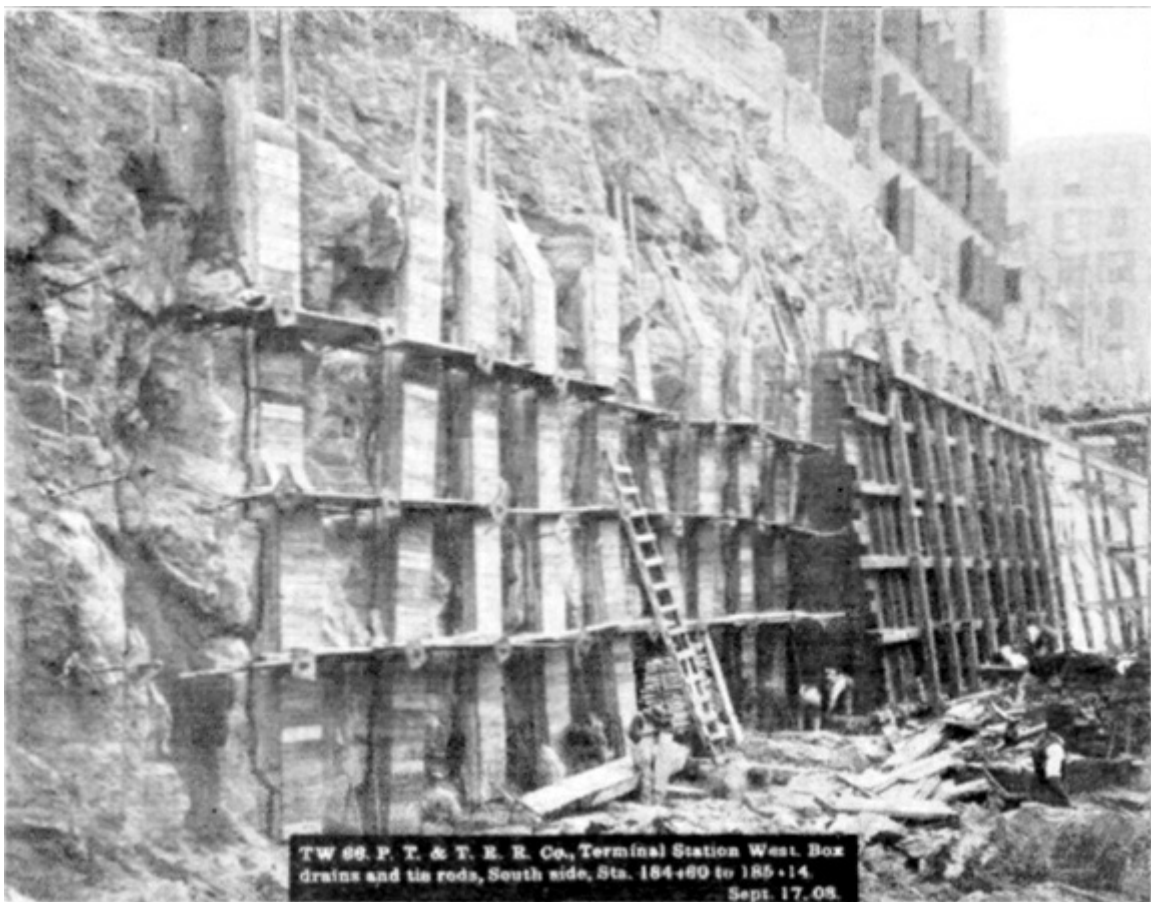
PLATE LI, FIG. 1.— TW 66, P.N.Y. & L.I.R.R. TERMINAL STATION WEST. BOX DRAINS AND TIE RODS, SOUTH SIDE, STA. 184+80 TO 185+14. SEPT. 17, 08.
