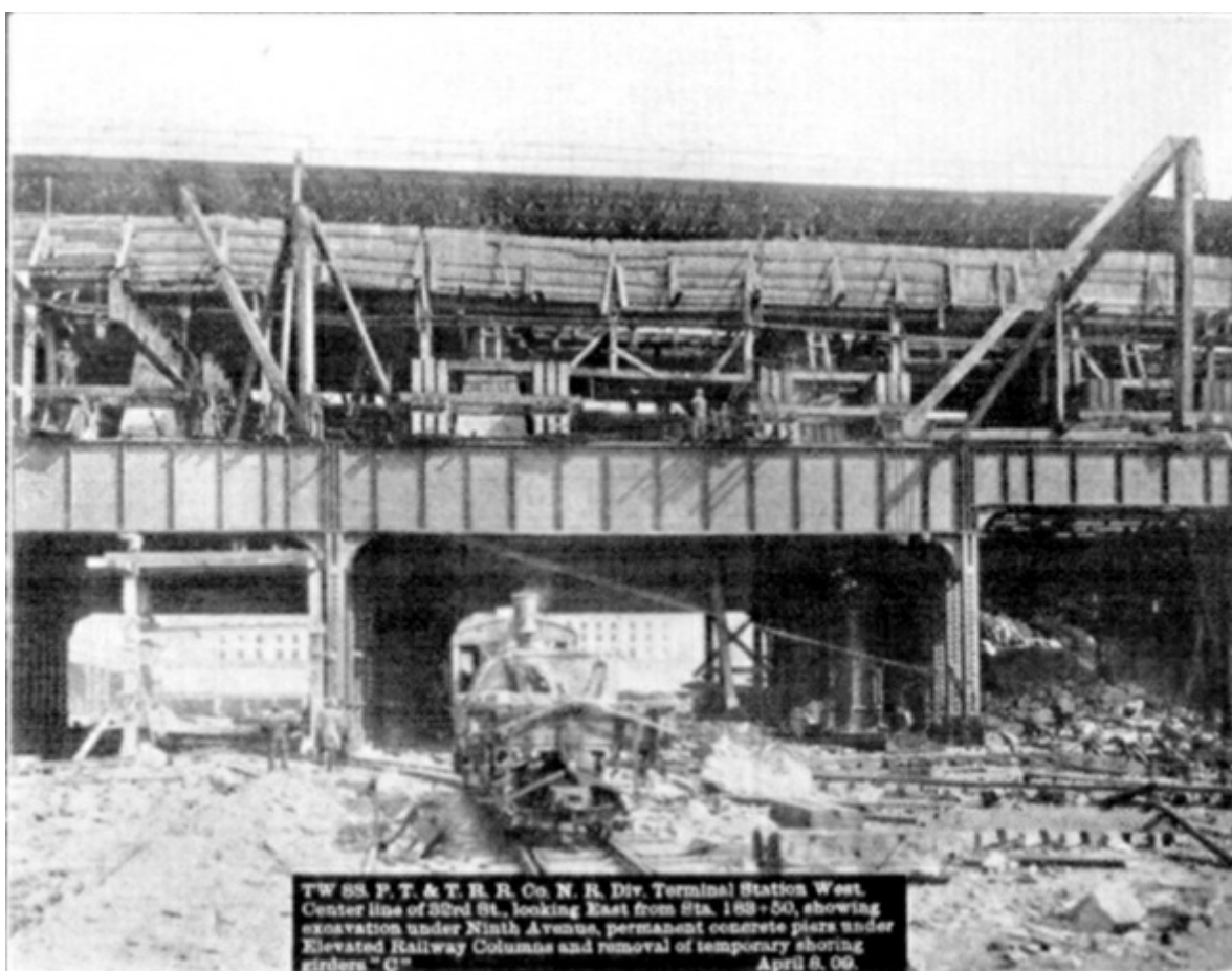
PLATE XLIX, FIG. 3.— TW 88, P.T. & T.R.R. Co. N.R. DIV. TERMINAL STATION WEST. CENTER LINE OF 32ND ST., LOOKING EAST FROM STA. 183+50, SHOWING EXCAVATION UNDER NINTH AVENUE, PERMANENT CONCRETE PIERS UNDER ELEVATED RAILWAY COLUMNS AND REMOVAL OF TEMPORARY SHORING GIRDERS "C". APRIL 8, 09.
