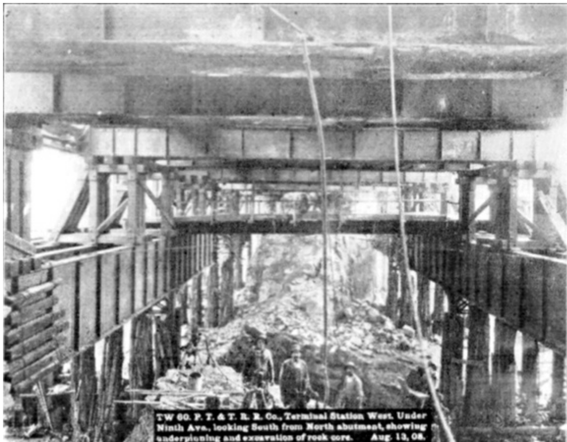
PLATE XLIX, FIG. 1.— TW 60, P.T. & T.R.R. CO. TERMINAL STATION WEST. UNDER NINTH AVE., LOOKING SOUTH FROM NORTH ABUTMENT, SHOWING UNDERPINNING AND EXCAVATION OF ROCK CORE. AUG.
