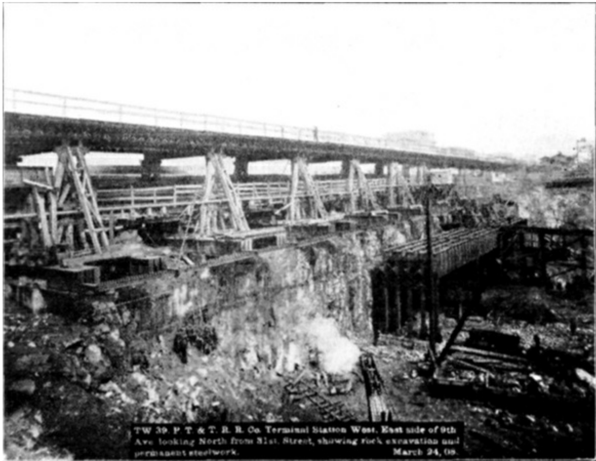
PLATE XLVIII, FIG. 2.— TW 39, P.T. & T.R.R. Co. TERMINAL STATION WEST. EAST SIDE OF 9TH AVE. LOOKING NORTH FROM 31ST STREET, SHOWING ROCK EXCAVATION AND PERMANENT STEEL WORK. MARCH 24, 08.
