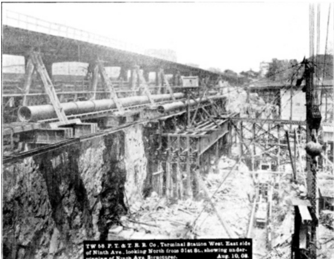
PLATE XLVIII, FIG. 4.— TW 58, P.T. & T.R.R. Co. TERMINAL STATION WEST. EAST SIDE OF NINTH AVE. LOOKING NORTH FROM 31ST ST., SHOWING UNDERPINNING OF NINTH AVE. STRUCTURES. AUG. 10, 08.
