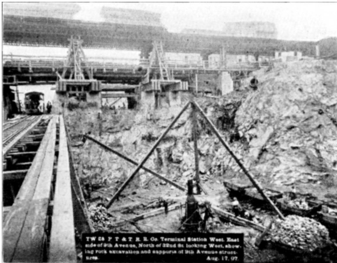
PLATE XLVII, FIG. 4.— TW 28, P.T. & T.R.R. CO. TERMINAL STATION WEST. EAST SIDE OF 9TH AVENUE, NORTH OF 32ND ST. LOOKING WEST, SHOWING ROCK EXCAVATION AND SUPPORTS OF 9TH AVENUE STRUCTURES. AUG. 17, 07.
