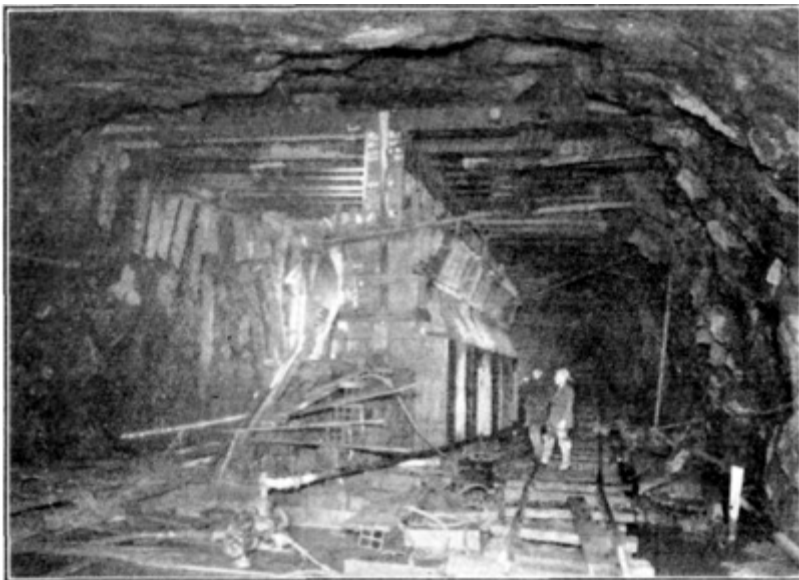
PLATE LX, FIG. 2.—CENTER WALL AND SKEWBACK UNDER I-BEAMS, AFTER REMOVAL OF DOUBLE ROW OF POSTS.
