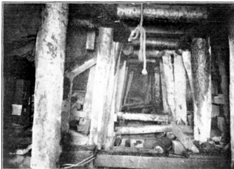
PLATE LIX, FIG. 2.—TIMBERING IN TOP HEADINGS ABOVE I-BEAMS.
