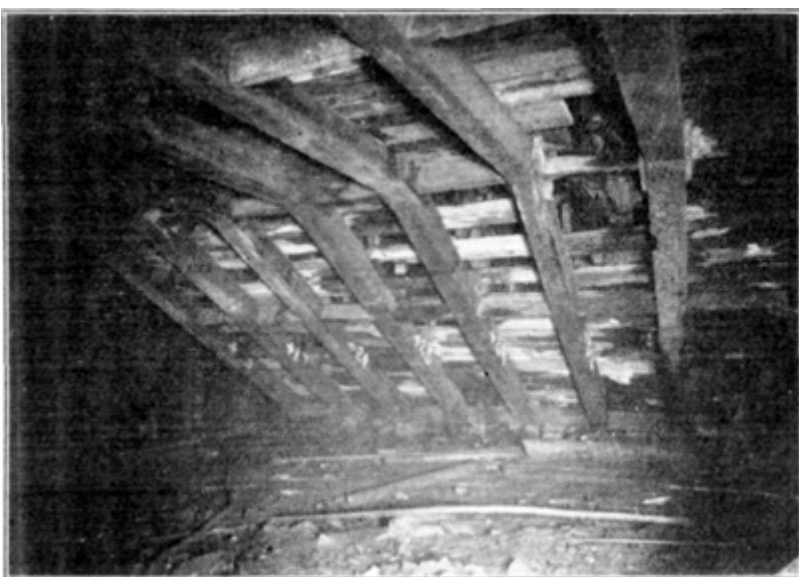
PLATE LX, FIG. 3.—TIMBERING IN FULL-WIDTH HEADING OF THREE-TRACK TUNNEL.
