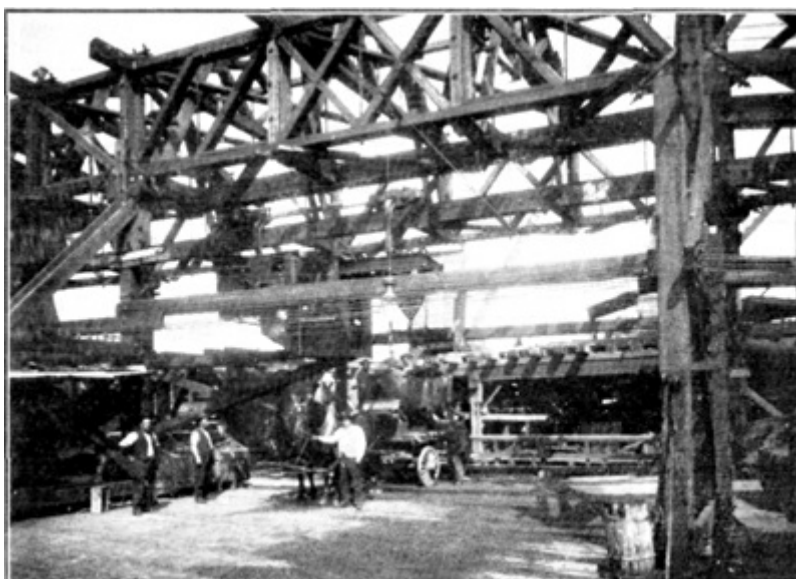
PLATE LVIII, FIG. 2.—TELPER STRUCTURE AND LOADING PLATFORM, FIRST AVENUE SHAFT.
