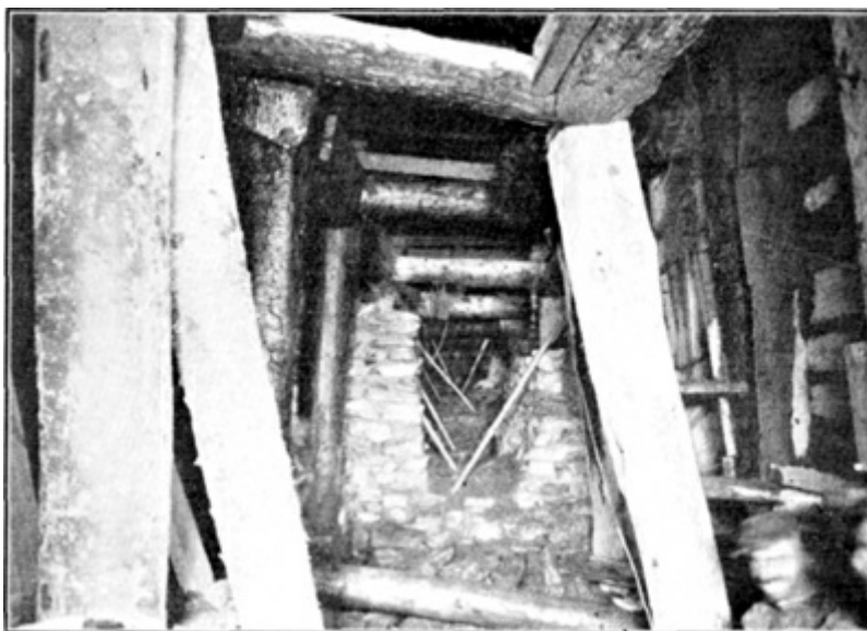
PLATE LIX, FIG. 4.—TIMBERING AND RUBBLE MASONRY OVER I-BEAMS.
