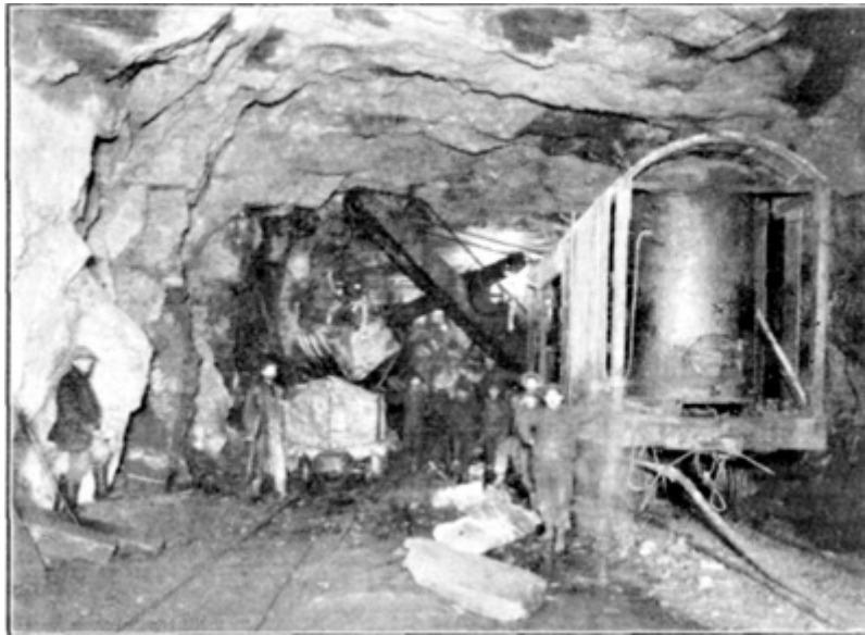
PLATE LIX, FIG. 1.—AIR-OPERATED STEAM SHOVEL USED IN TUNNEL.
