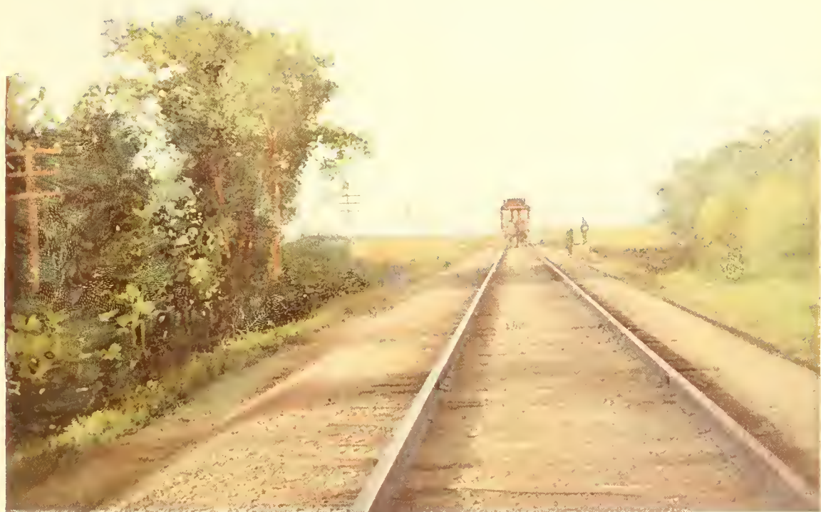
MAIN LINE OF UNION PACIFIC, WOOD RIVER, NEB., Ballasted with the Famous Sherman Gravel.
